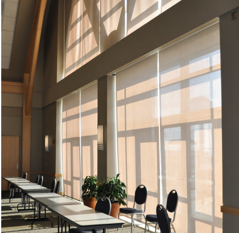
THIS PAGE: Three views of the Davis student center on the University of Vermont campus in Burlington. Featuring blackout shades behind sheer shades on a massive 30-foot wide window, the Gordon's team had to use cantilever lifts to reach to uppermost portions in what was a very tight-fitting installation. Two motors were installed to manage the shades.
